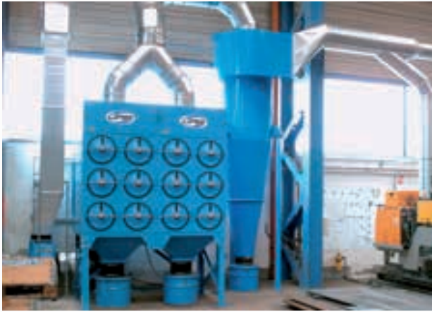
for plasma cutting table, here with pre-separator (cyclone)
